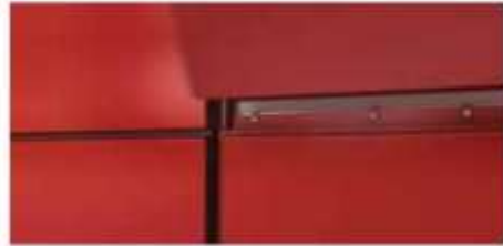
Subsequent cassettes hook into neighbour, next layer fixes into lower layer and neighbours.
