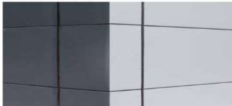
System Q2A with Epdm gasket with an aluminium insert
